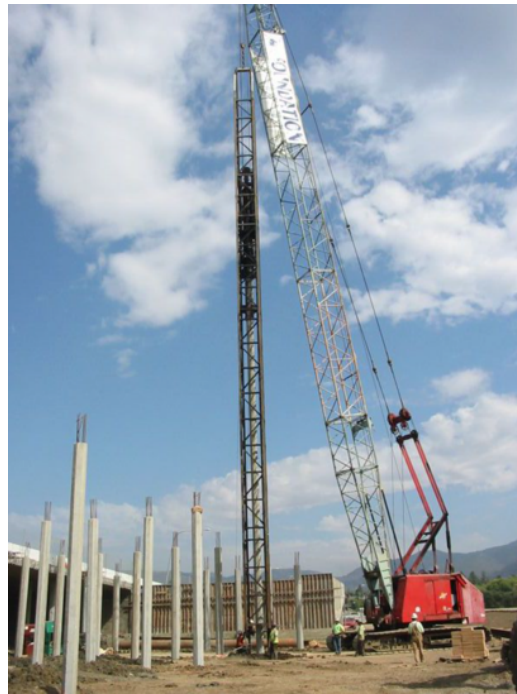
Figure 2 – typical driven concrete piles pitched using a crane and hammer (photo copyright: Argyriou https://tinyurl.com/yc4a4v8x ,)
